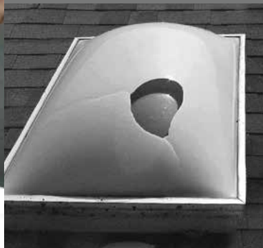
Old acrylic domes can be easily damaged.
